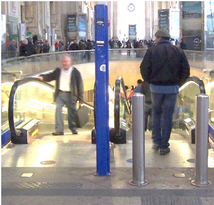
Sloped people mover is more universal than escalator Milan Central Station, Italy
