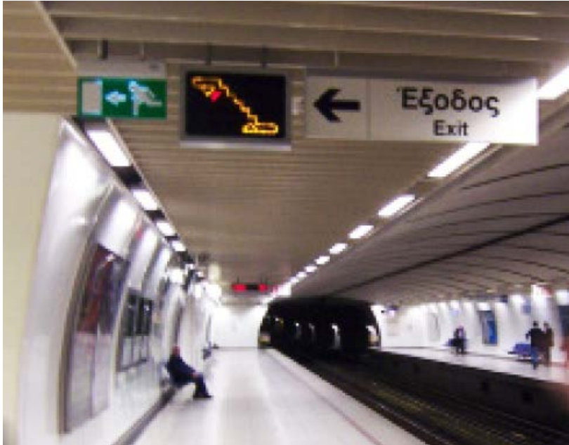
Real time escalator direction indicator Athens Metro, Greece
