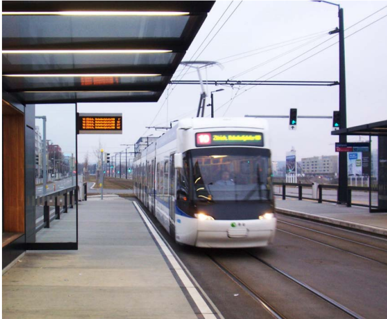
A light rail station
