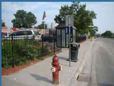
Chicago Avenue at Franklin Avenue
