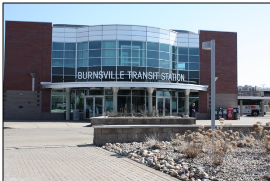
Burnsville Transit Station
