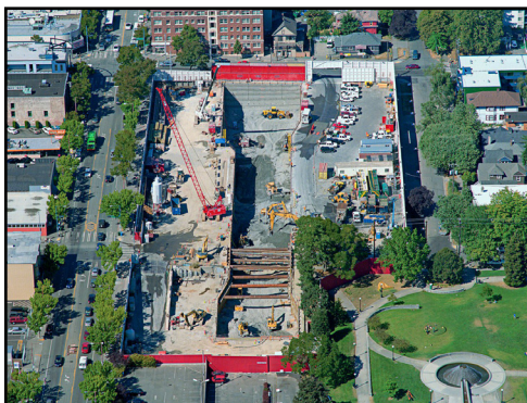
Capitol Hill Light Rail Station, during construction. Seattle, WA
