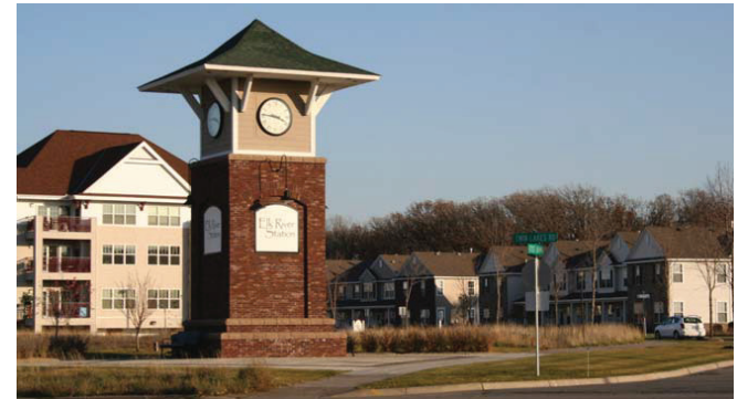
Elk River Transit Station with residential buildings
