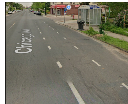
Figure 30 Example of a bus bike mixing zone on Chicago Ave S at E 32nd St.
