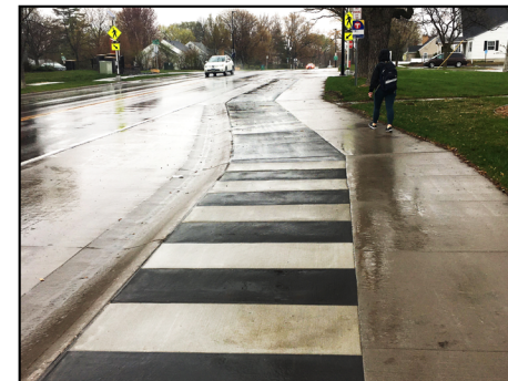
Figure 34 An example of a shared bus stop on Cedar Lake Rd at Hampshire Ave S in St. Louis Park
