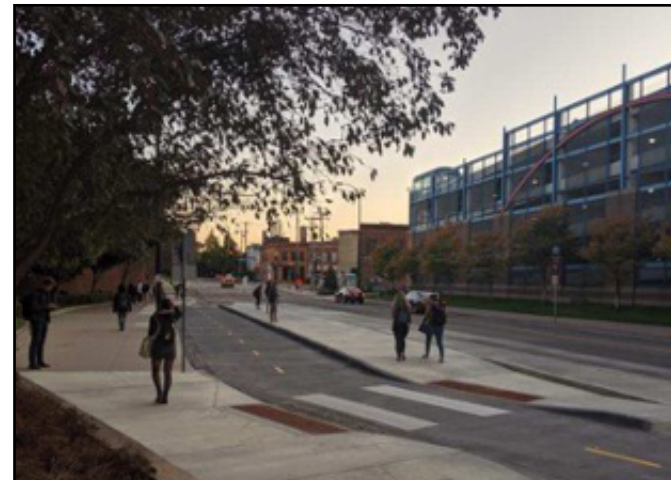
Figure 32 A floating bus stop on the University of Minnesota Twin Cities campus
