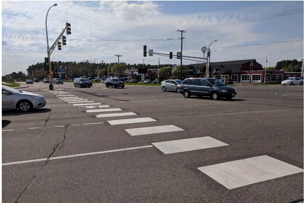
Highway 61 at County Road E (Facing Northwest)
