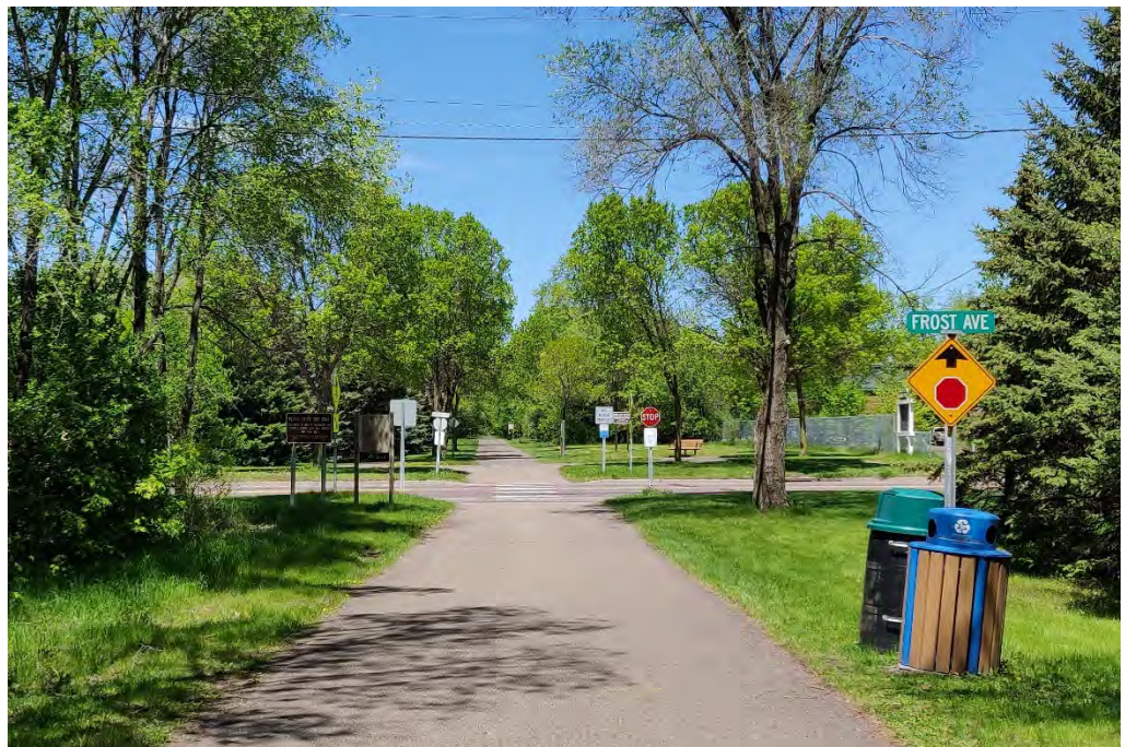
Ramsey County Rail Right-of-Way at Frost Avenue (Facing North)
