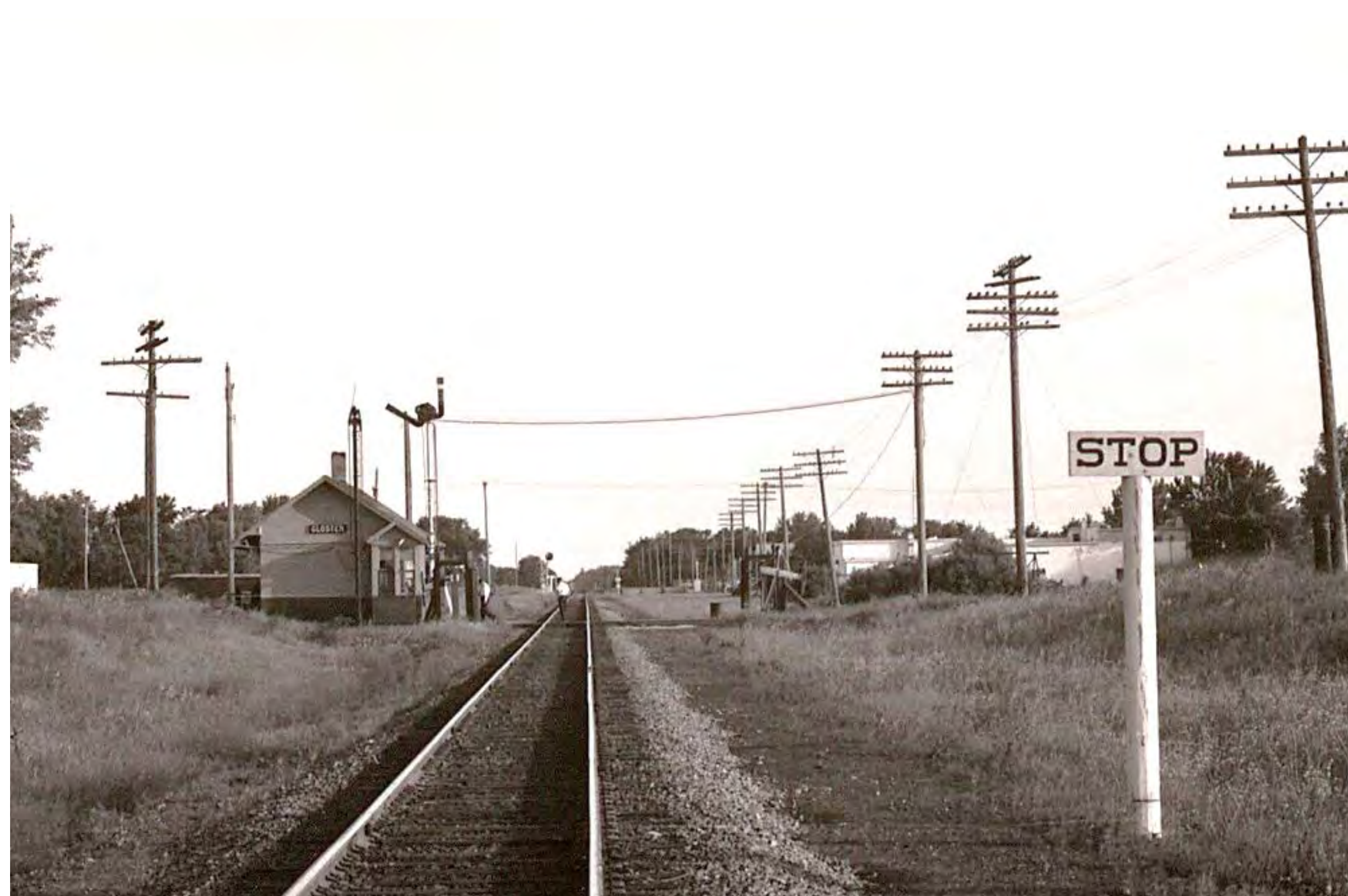
NP track looking south toward Gloster Junction, 1963 (Lake Superior and Mississippi Railroad Historic District)
