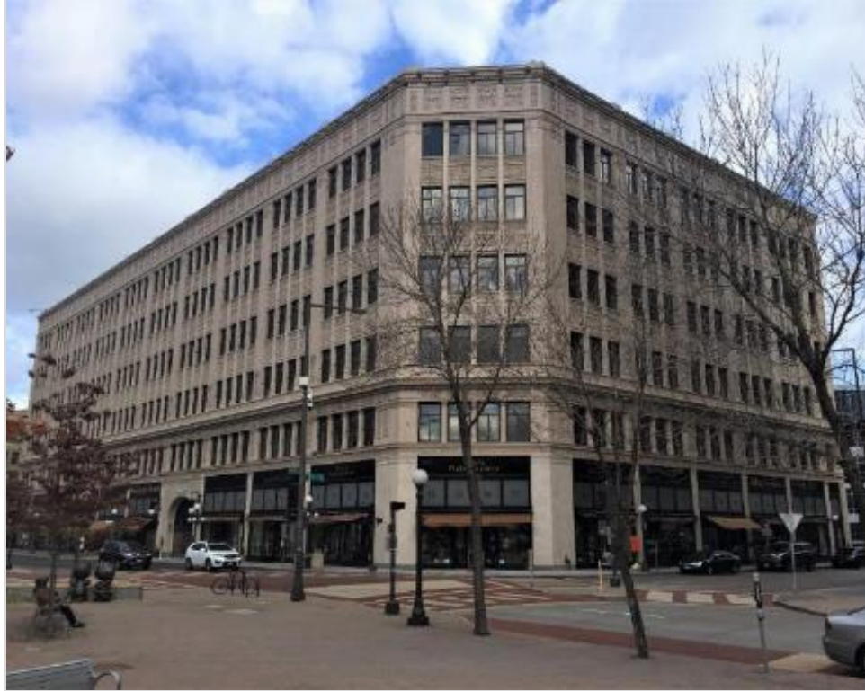
Figure 75. Hamm Building, facing north-northeast.
