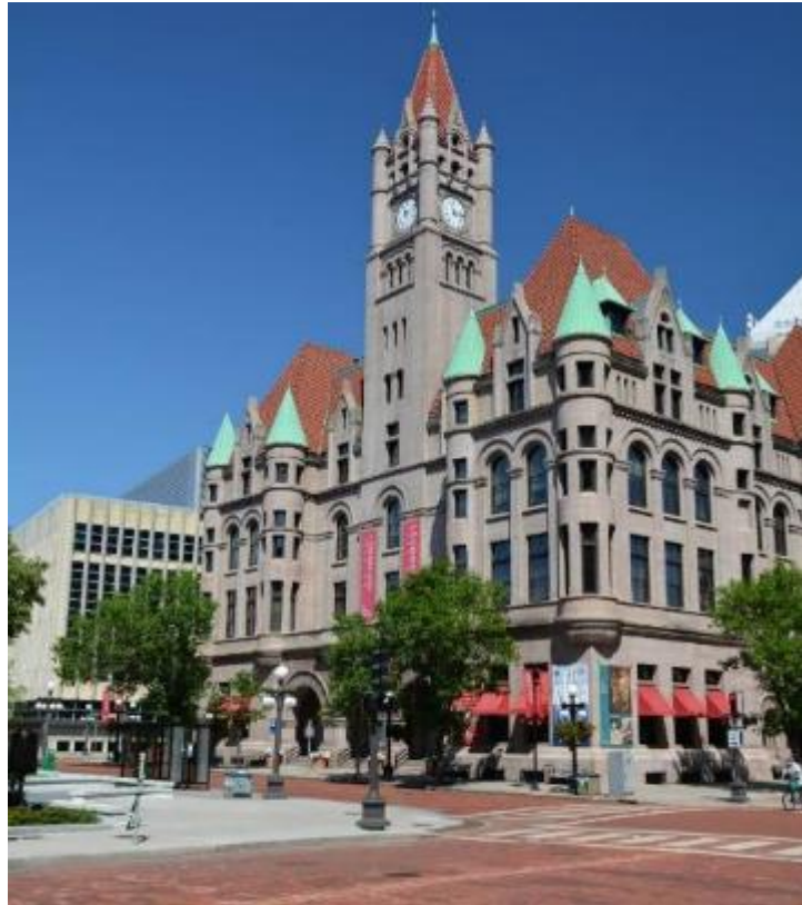
Figure 67. Landmark Center, facing north-northwest.
