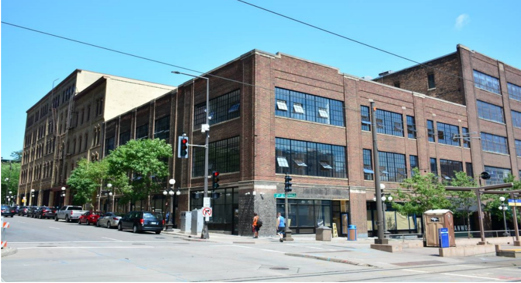
Figure 40. LHD, View of the Samco Sportswear Building (contributing) at the corner of 4th and Sibley Streets, facing northeast.
